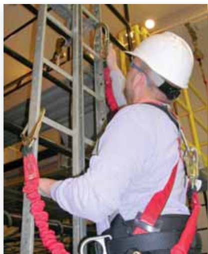
Climbing with a twin-leg Diamond Shock-Absorbing Lanyard
