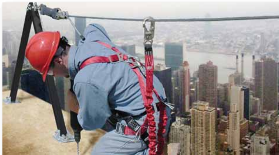
A Diamond Shock-Absorbing Lanyard used with the SkyLink Horizontal Lifeline
