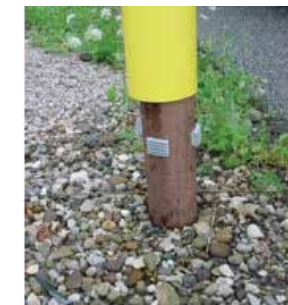
Step 2 - Place cover over grip tabs.
