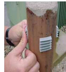
Step 1 - Install self-adhesive grip tabs.
